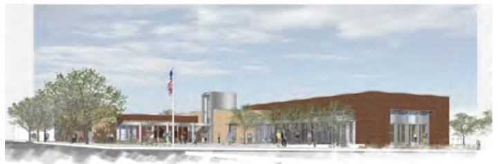
Above, a view of the community center from Maryland Avenue.
